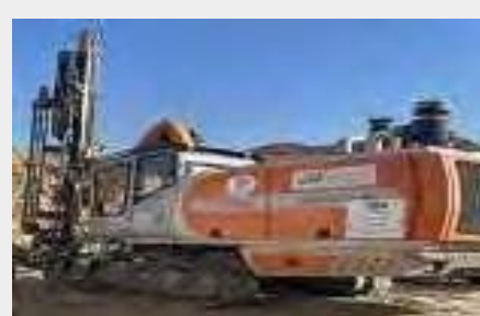
DRILLING MSCHINE NOS 2
